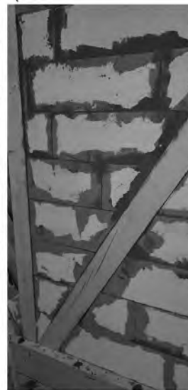
Type 5 – AAC masonry infill
