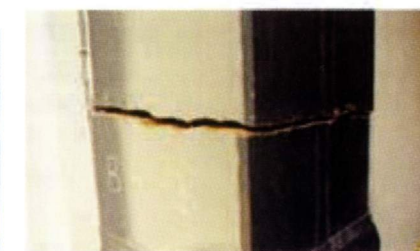
Brittle Fracture in Kobe Earthquake
