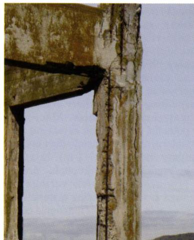
Deterioration of RC building in the coast of a bay
