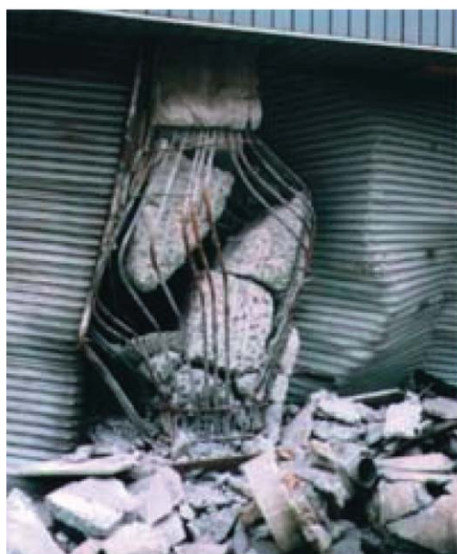
阪神・淡路大震災で実際に起きた柱のせん断破壊 Damage from earthquake
