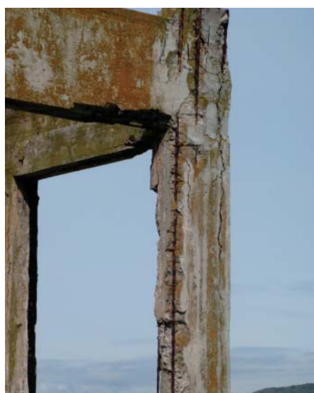
湾岸コンクリート造建物の劣化 Deterioration of reinforced concrete buildings in bay area
