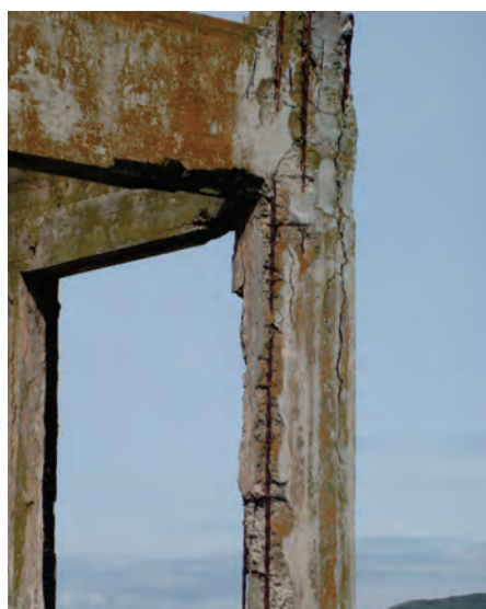
湾岸コンクリート造建物の劣化 Deterioration of reinforced concrete buildings in bay area
