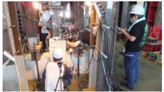
Damage evaluation based on crack pattern and its width on the concrete foundation of exposed column base
